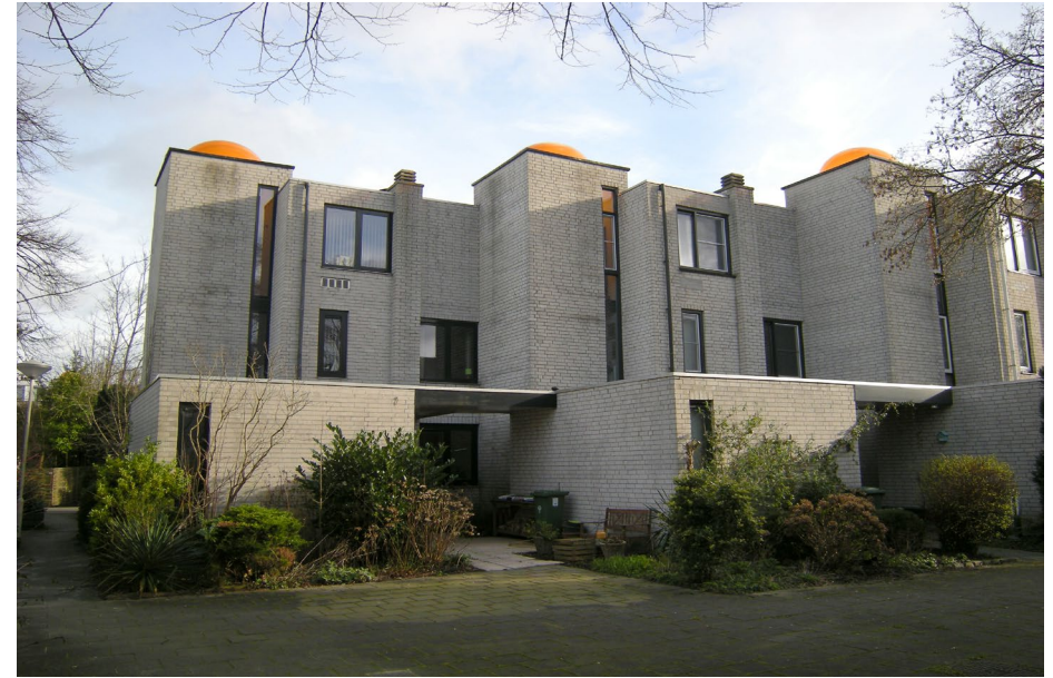
Koepeltjeswoningen van architect Benno Stegeman, 2019 [Contrei]
